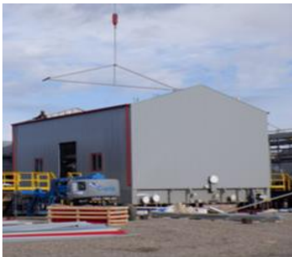
Compressor Buildings Installed
