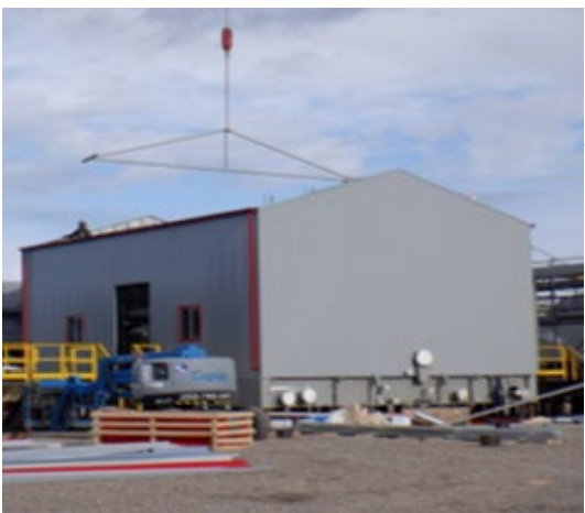
Compressor Buildings Installed
